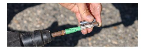
Drill all holes to the depth indicated by the tape or marker applied to the drill in step 4. Holes must be vertical to properly anchor the bike rack.
