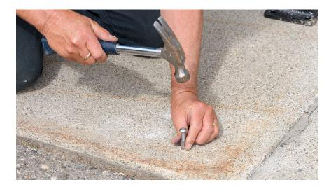
Fix the anchors in place with the supplied set tool and a hammer to expand the base of the anchors and permanently secure them to the pad.
