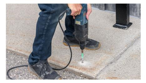
Vacuum (or blow) the drilling dust and debris to leave a clean hole. A screwdriver can be useful to loosen any debris in the hole.
